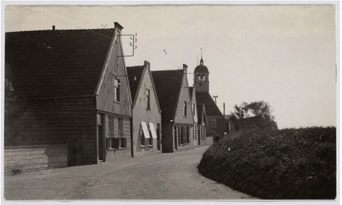
Durgerdammerdijk B 55- B 66
